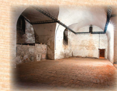
Under the church there is a spacious crypt, for the construction of which the Trinitarians used a deep trench around the Upper Castle, together with the older masonry structures of the Castle. They fully used the terrain for making a crypt under the entire church. It is the burial place of some of the members of the order, people who donated to the church and local nobility.
